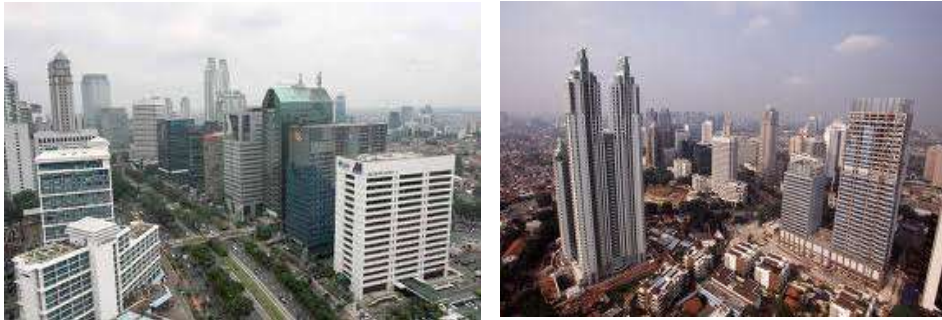
Figure 2 Densely spaced buildings.
