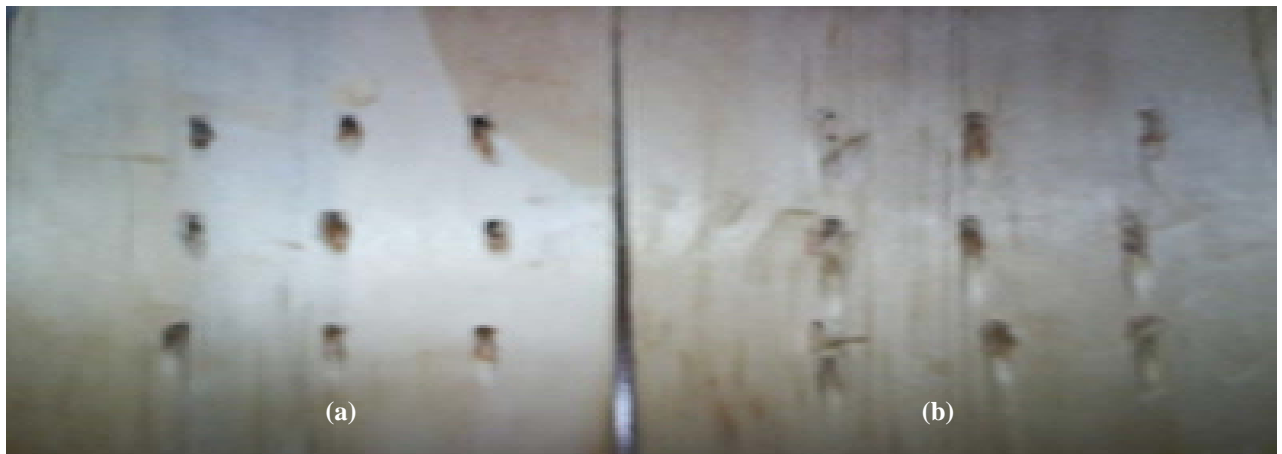
Figure 14. Damage on the inside surface of plywood side plate, (a) sengon -plywood (b) meranti -plywood
