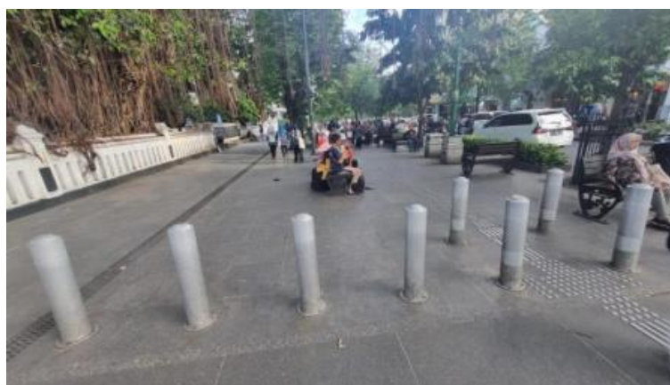
Figure 2. Malioboro Street's Safety Curb as a Barrier for Wheelchair Users
