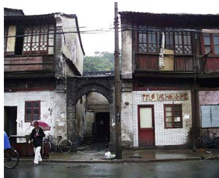
Fig.5 Dilapidated buildings before the project
