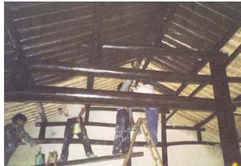
Fig.9 The work of remedying architectural components
