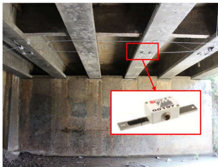
Figure 1 B-WIM instrumentation on the PCI girder bridge.
