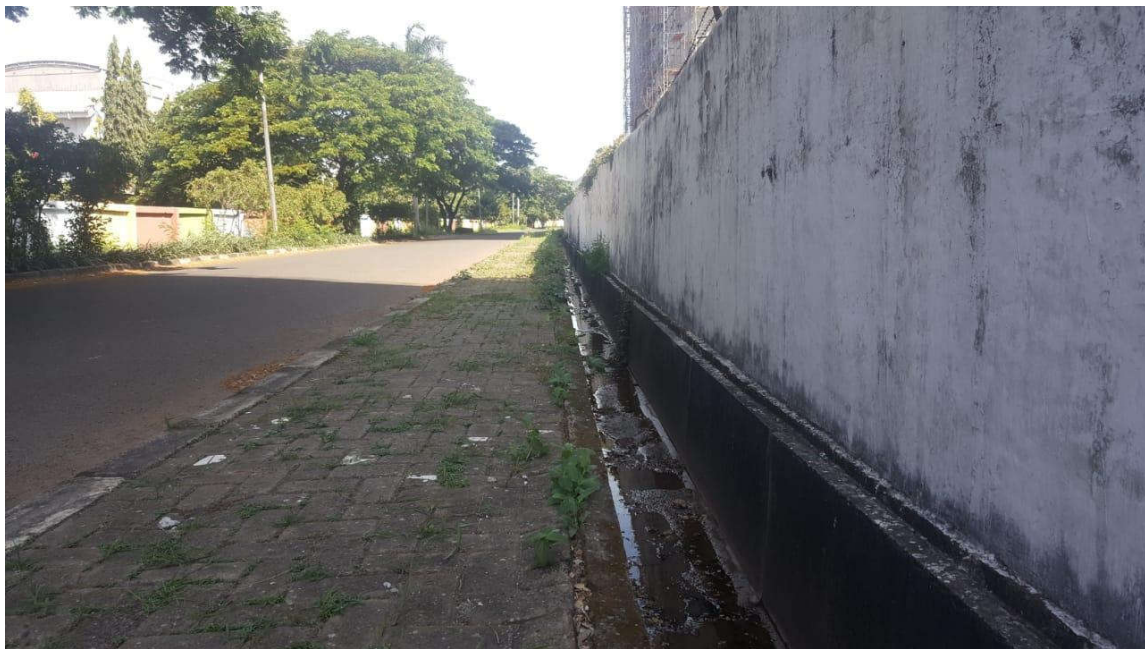
Figure 4 City drainage channel at the west perimeter of the project area.
