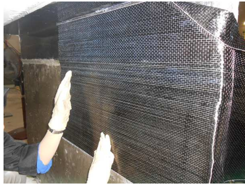
Figure 4 Repair and retrofitting process of test model using CFRP fabric.
