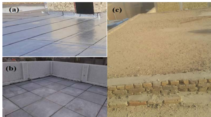
Figure 5 Popular roofing materials used: (a) Ezukam, (b) concrete tiles, (c) clay.
