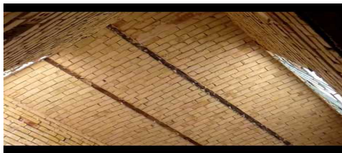
Figure 2 Fired clay brick roof (jack arch ceiling).
