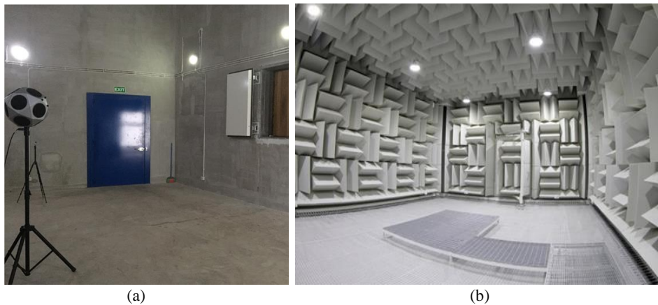
Figure 3 Sound insulation chamber (SIC) located in the Center for Advanced Science (CAS), Bandung Institute of Technology (ITB): (a) reverberation chamber, (b) anechoic chamber.
