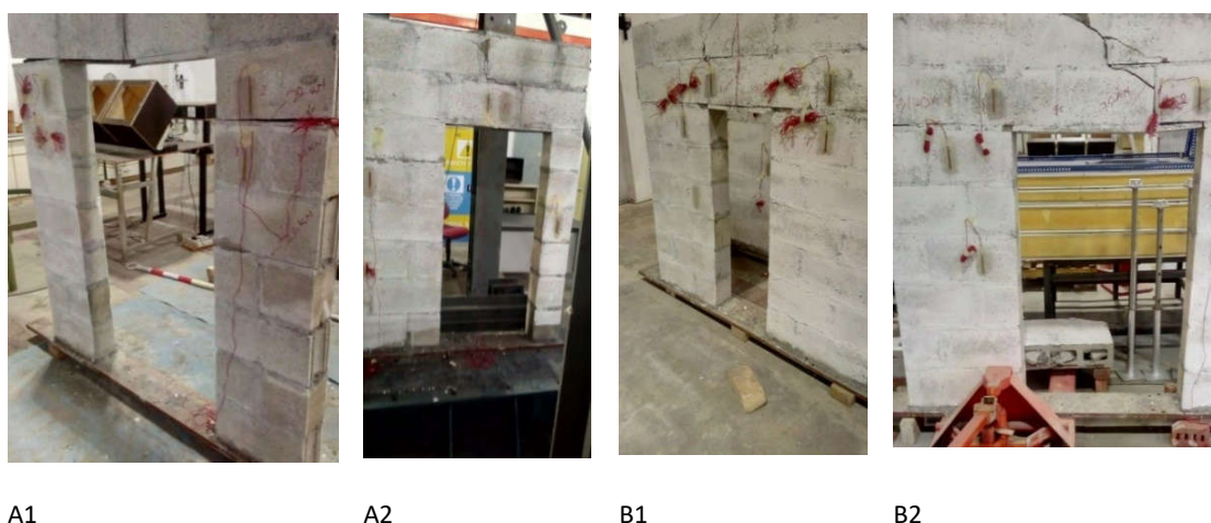
Figure 3 The cracking patterns of wall panels A1-B2.
