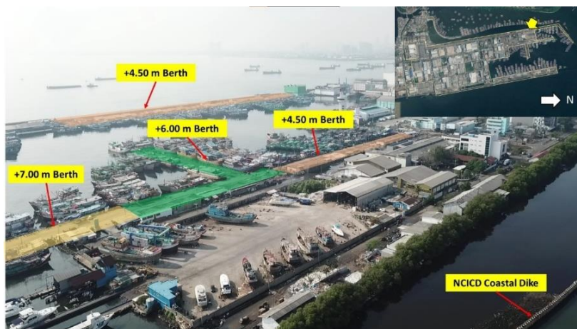
Figure 3 Elevations of existing berths. The yellow arrow in the inset indicates the viewing perspective.
