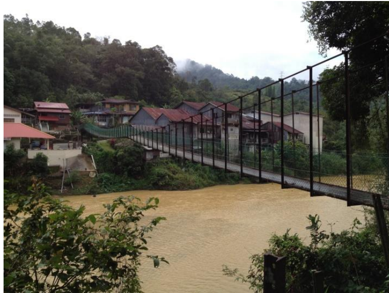
Figure 5. Kolong Pahat hanging bridge.
