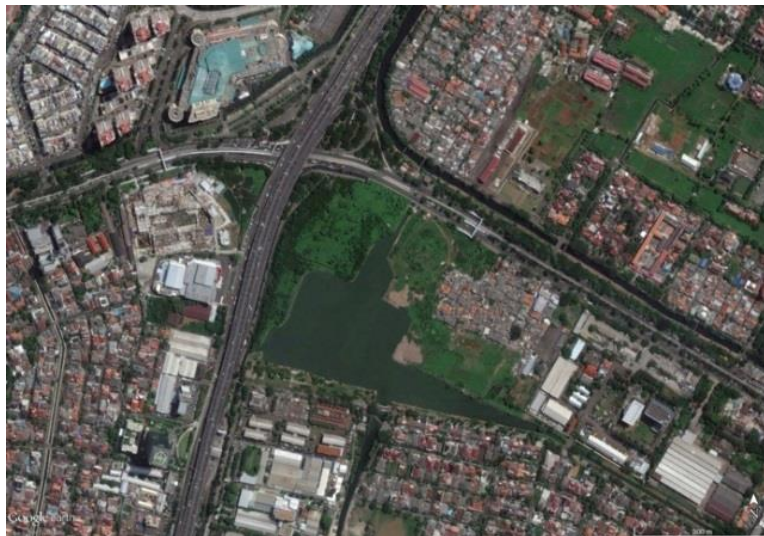
Figure 15. Waduk Ria Rio after works carried out. Source: Google Earth (2018).
