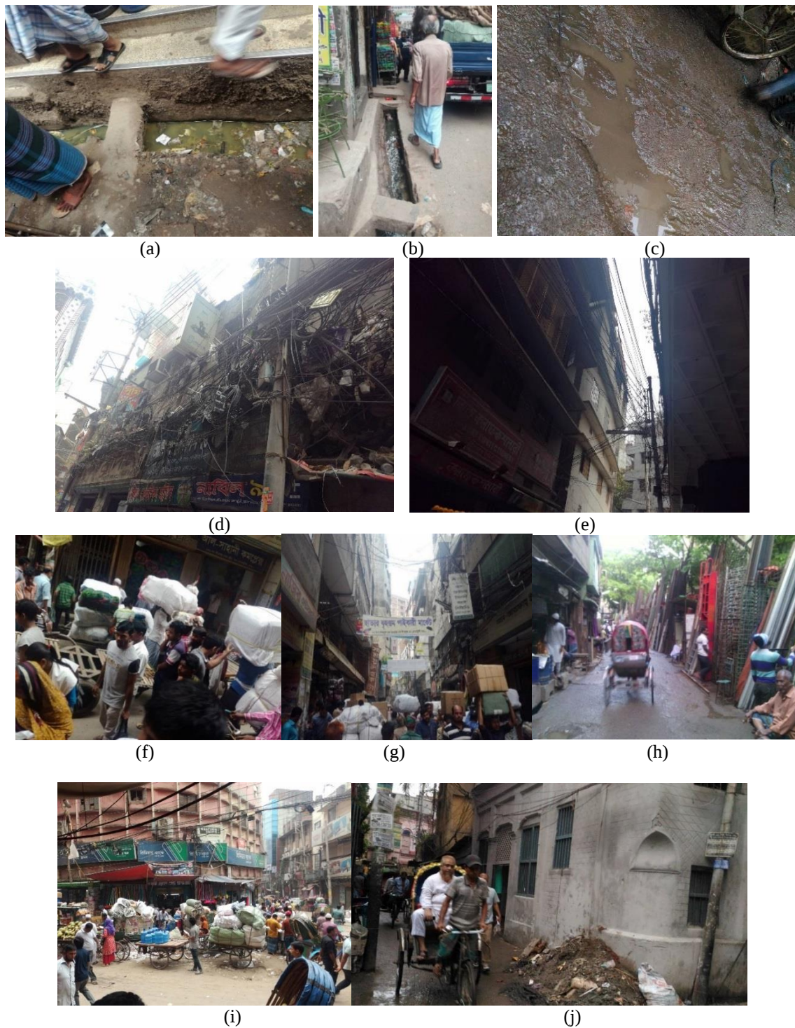
Figure 8 (a), (b), (c): Poor drainage (d), (e): unsafe, earthquake-prone and hazardous buildings and road conditions, (f),(g) narrow and (h) hazardous roads. (i), (j): Uncovered bins and open dumping of waste. (Source: author)
