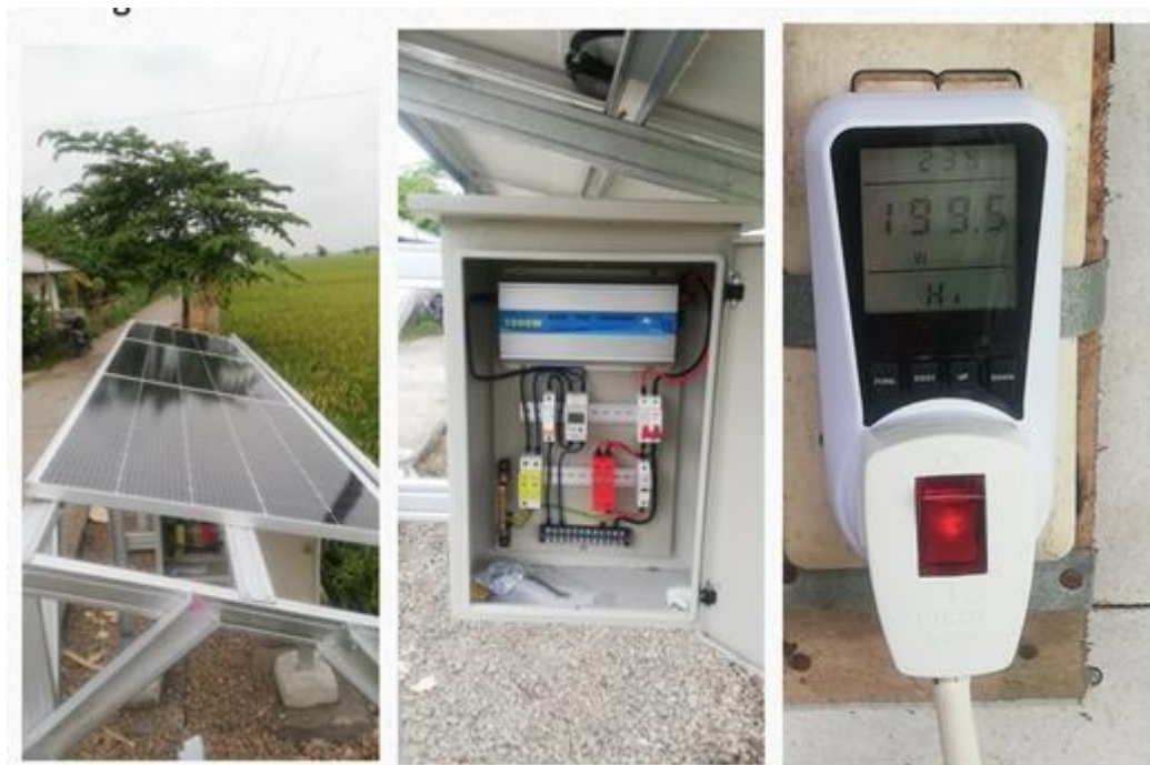
Figure 3. Solar panels supported by light steel frames (left); inverter, circuit breakers, surgearrester installed in panel box (middle); Watt meter for monitoring the generated power at any time (right).
