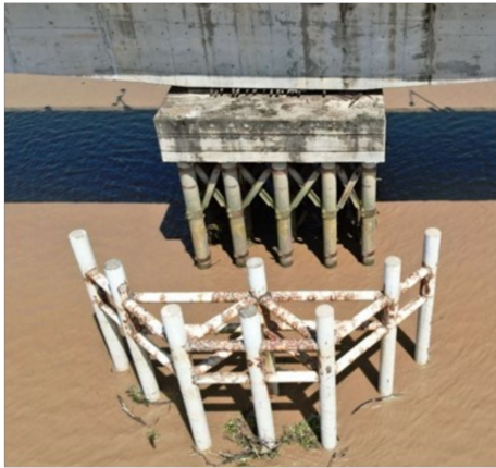
Figure 1. Bracing in pedamaran II bridge foundation
