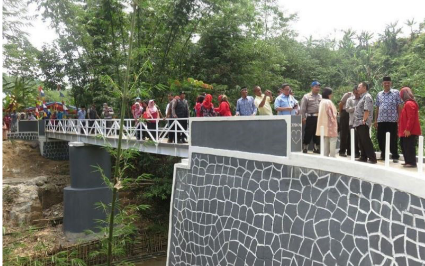
Figure 1. Jembatan Hati 3 (Source. Personal Picture)
